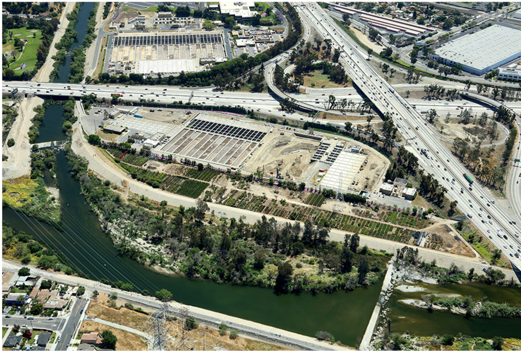
Figure 1-4. Aerial Photograph of LACSD's San Jose Creek East (SJCE) Plant.
