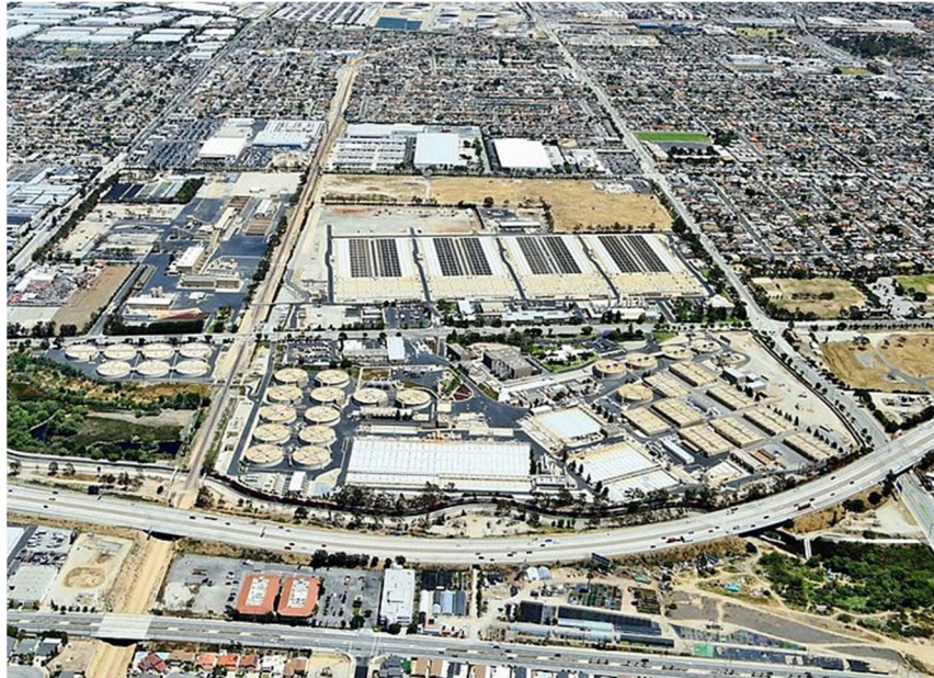
Figure 1-2. Aerial Photograph of JWPCP.
